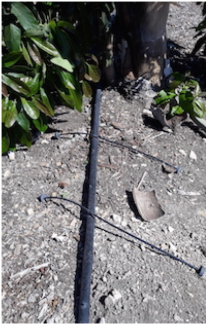
Mature trees have 8 emitters each; others vary given the tree's size and age
