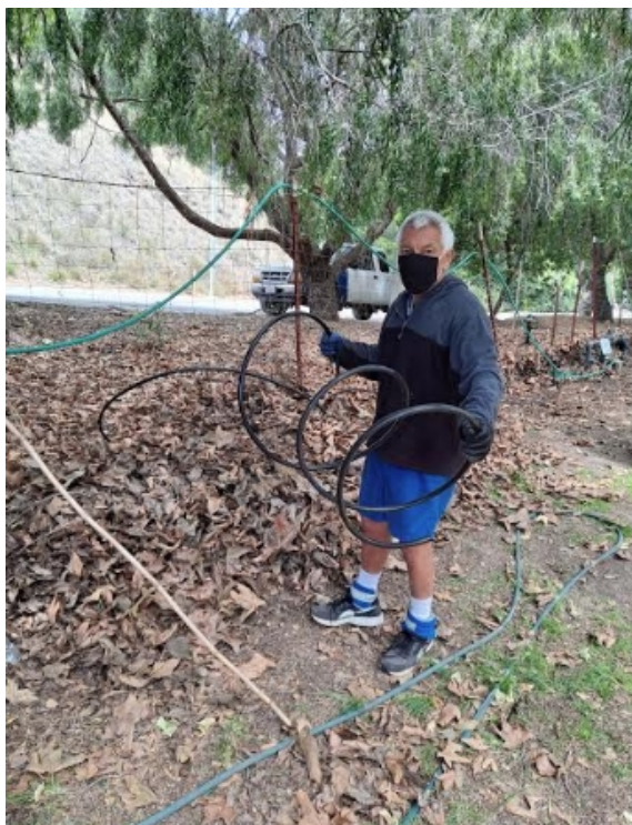
Manny uncoils the drip line tubing.
